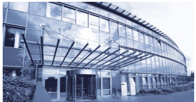
Basler AG Germany, Headquarters
